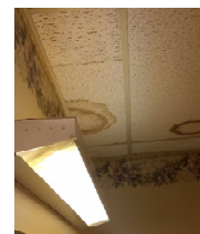
Ladies Room Light/Ceiling
